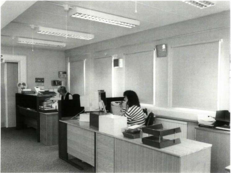
Figure 16 Natural lighting is blocked out and replaced by artificial lighting to avoid glare
